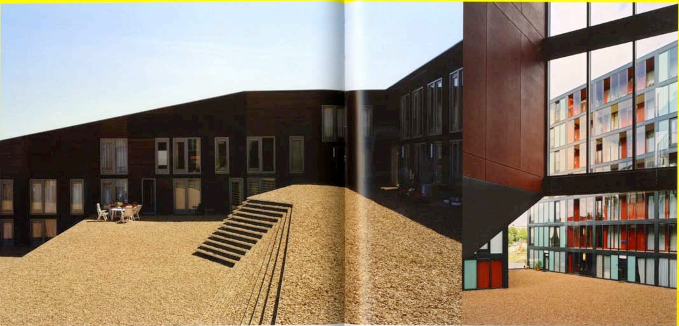
> Schöta 1 and 2 , Clinge Terrace, Dordrecht, the Netherlands, 1997-2002; (left) sloped landscape and terraces of Schöta 2
